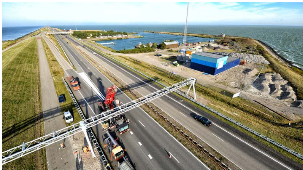
The Blue energy pilot plant located on the Afsluitdijk. The pipe passing over the road serves to transport the salty seawater from the Waddensea to the plant.
